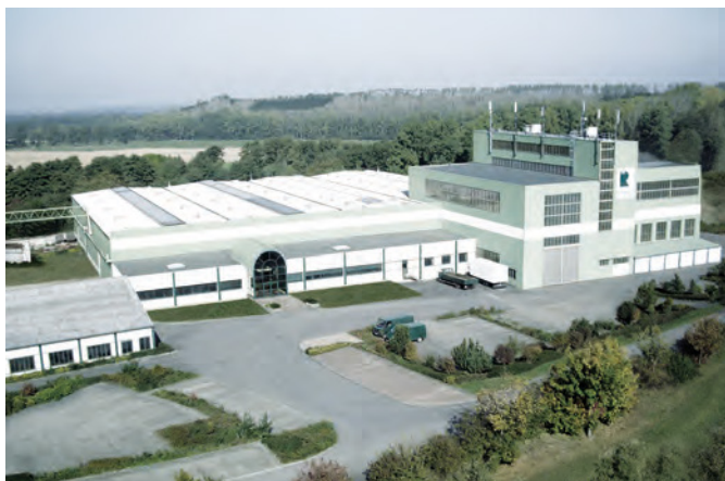
Richter Plant I pulp & reject in Hürtgenwald
